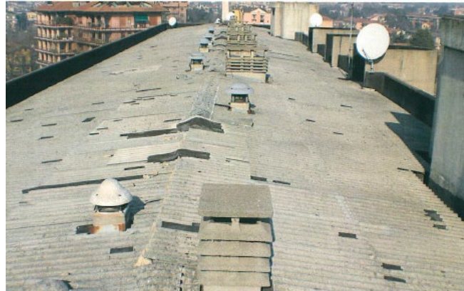
Figure 2 - Roof in asbestos cement before maintenance intervention
