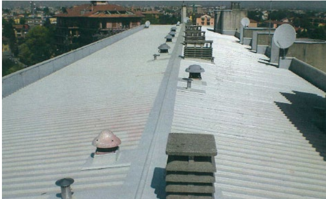
Figure 3 - Roof after the maintenance intervention
